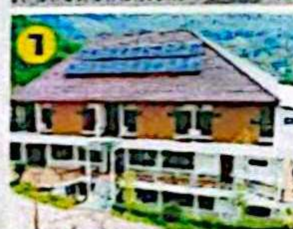
Solar Home System On Grid
